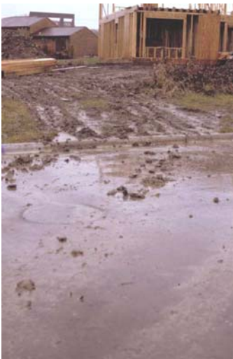
Tracking of sediment onto roadways leads to contamination of our lakes and streams.
