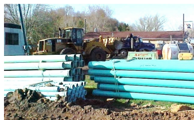
Constructing the Village of Melvina's collection system
