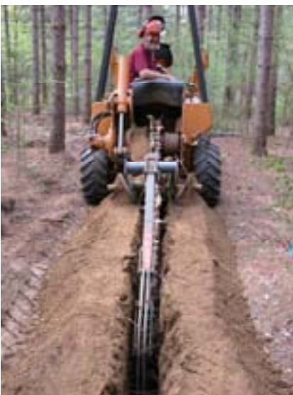
Roots are severed using a trencher
