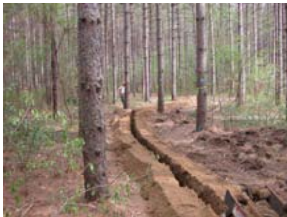
Right after the site is trenched.
